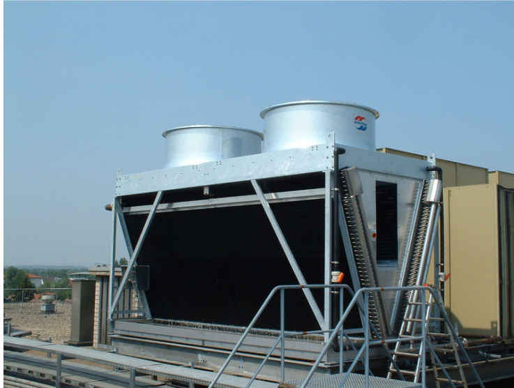
Hybrid condenser with desuperheater for Ammonia refrigeration in food industry
