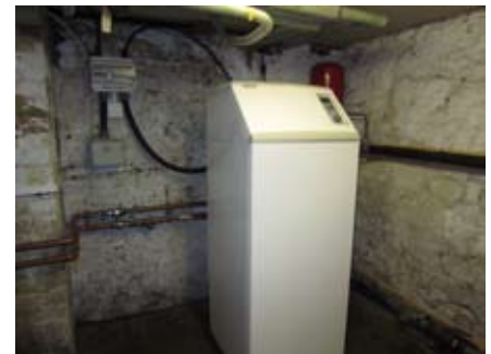
Heat pump during installation
