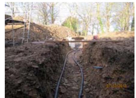
Ground works in progress
