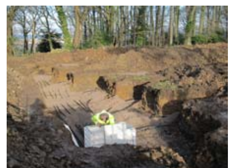
Building the manifold pit
