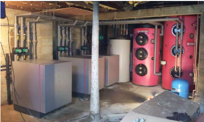
Three heat pumps in the plant room
