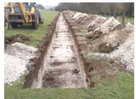
Horizontal collector array ground works in progress
