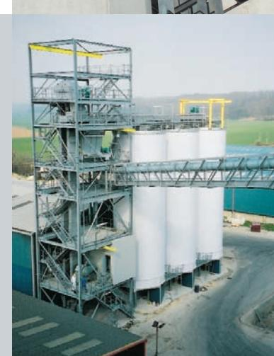
Our Bucket Elevators provide the power & efficiency required for large capacity work such as silo & bunker filling and other applications in excess of 80 meters vertical lift.
