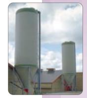
Silo diameter 2.4m Dome height 0.6m Cone depth 1.95m Cone angle 60°
