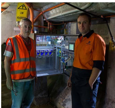
Scott MacDonald, Project Manager for Freyssinet with David Celine from Omniflex, during system commissioning.
