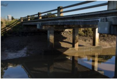
Cardinia Creek Bridge.
