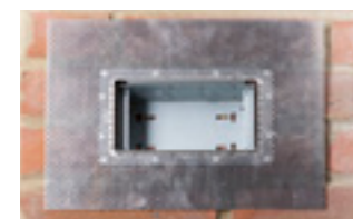
FIX WALL BOX AND PLASTER RING TO WALL
