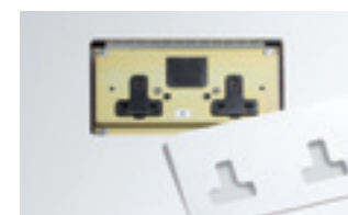
ADD FRONT PLATE ADJUST AND FINISH
