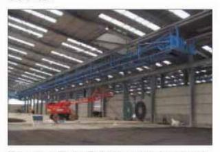
The unique Redler En-Masse principles inherent within the bridge conveyor provides for the automatic discharge of product across the full width of the store from floor level right up to the underside of the bridge conveyor. A high level probe within the bridge conveyor triggers the incremental and automatic movement to a new working position, thus storage is maximised over the full height and width of the store.
