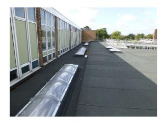
The works to Burscough Science College involved the application of 120mm insulation & a two layer, bituminous membrane, offering a 25 year guarantee.
