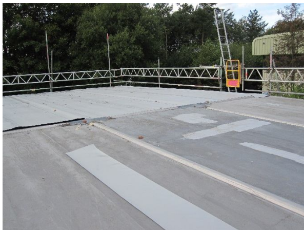
Preparation & installation works in progress
