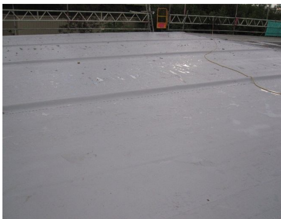
Completed roof works prior to scaffolding being removed
