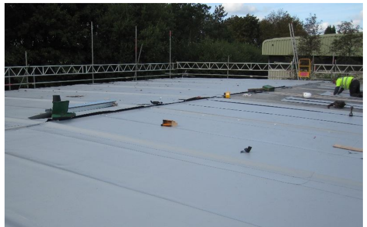
Areas of completed roof deck
