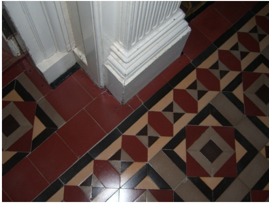
After with tiles restored, cleaned, holes filled & door threshold fitted.
