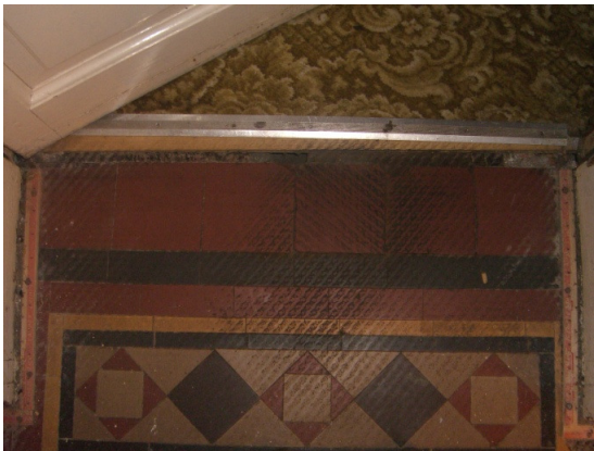
Before with loose tiles, paint & Dirt
