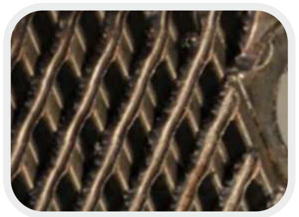
Cleaned primary water circuit
