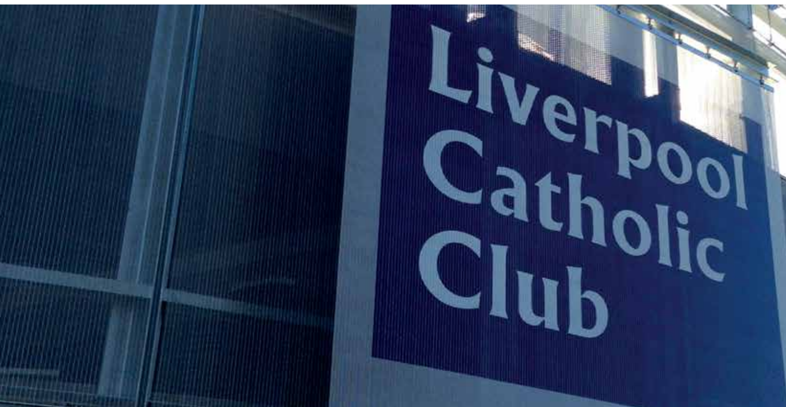
Mesh: Omega 1505 with screen print, project: Liverpool Catholic Club, Australia, architect: Wood & Day Partnership
