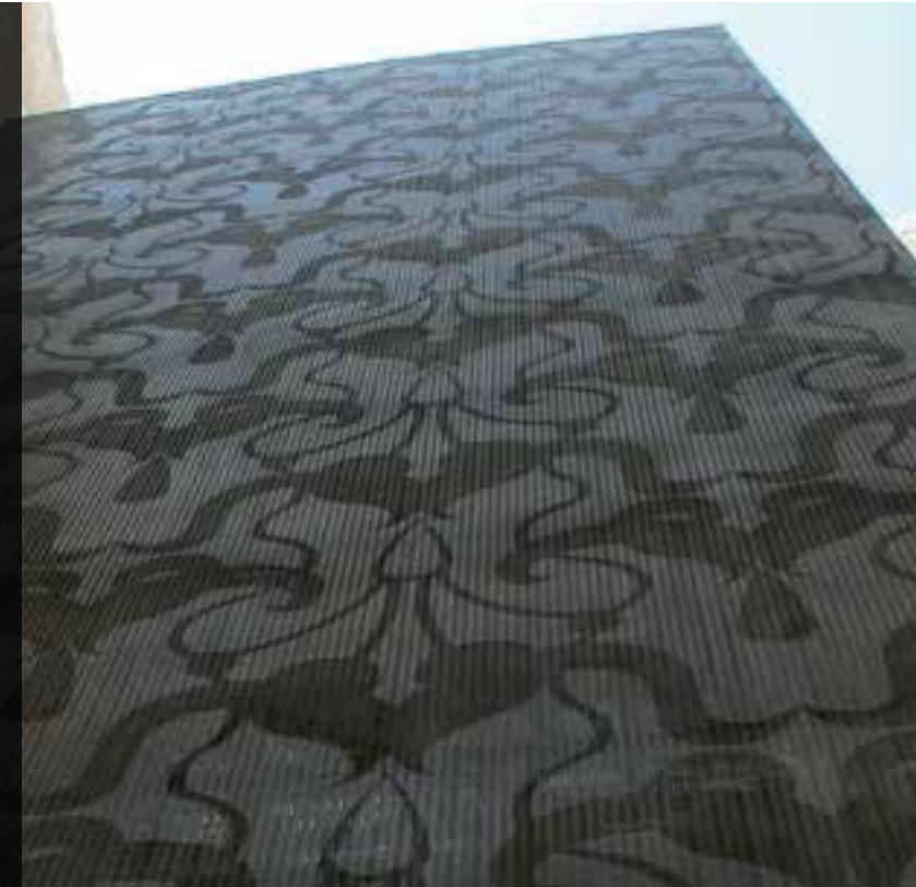
Mesh: Omega 1520 with blasted surface, project: Male & Female Student Housing, Qatar, architect: Treanor Architects
