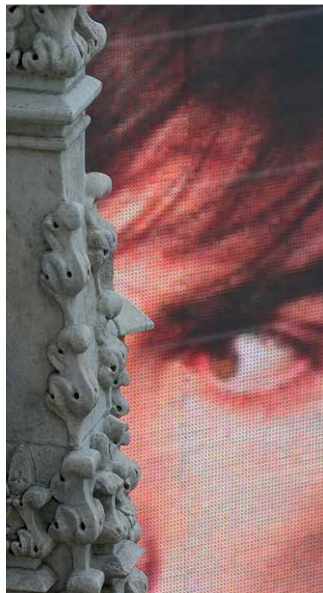
Mediamesh®: the LED density determines the resolution of the images (7)
