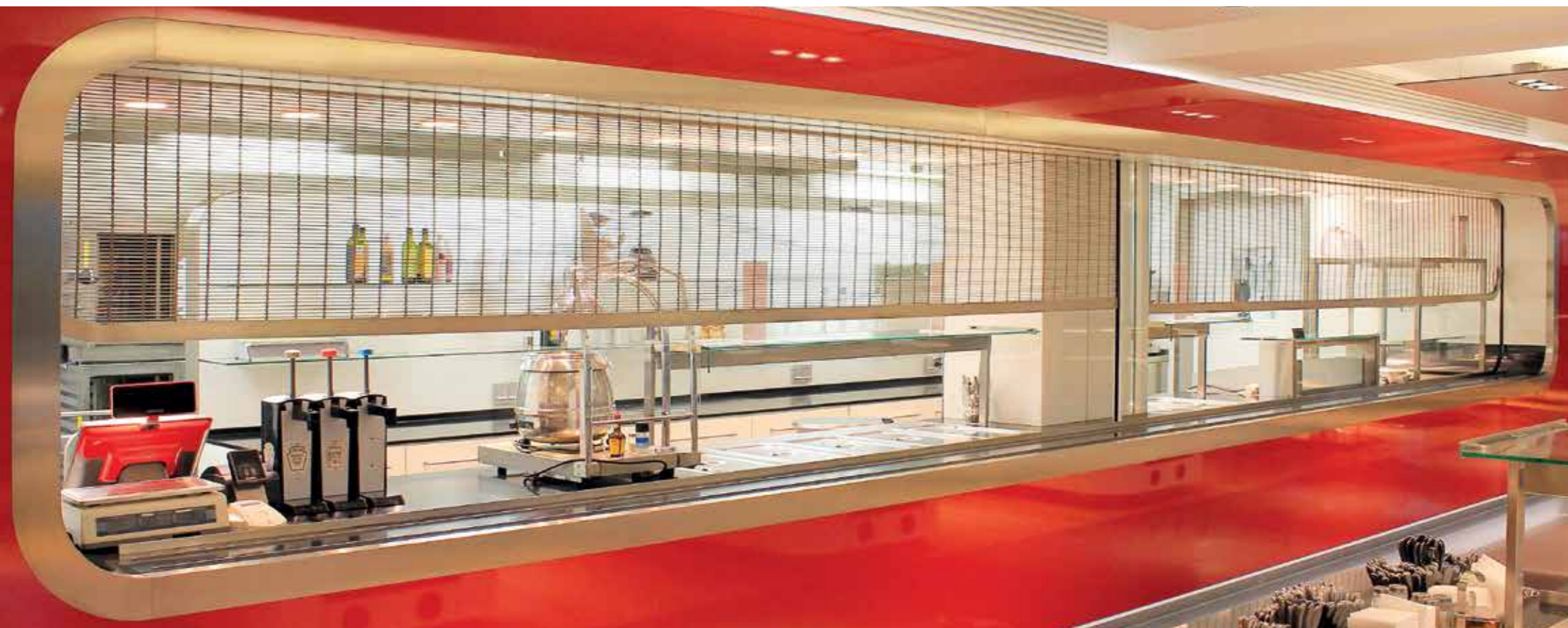
Roller shutter in a canteen, Münster, architect: Vervoorts & Schindler Architekten, Bochum, mesh: Tigris, ©GKD/Holtkötter
