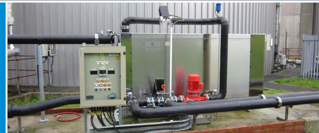
Turnkey Heat Exchanger with integral temperature and flow control installed for ▲ United Utilities
