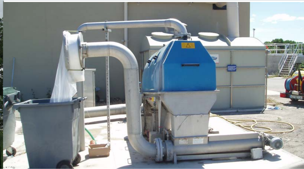
Roto-sieve Drum Screen and screenings handling equipment for liquid/solids separation ▲
