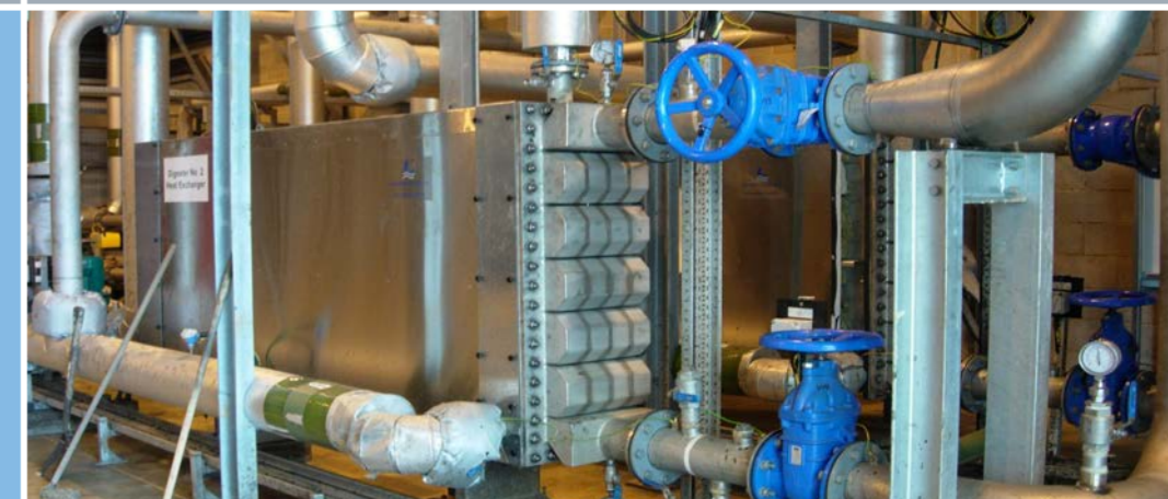
Sludge/Water heat exchanger installation at Kings Lynn for Anglian Water ▲
