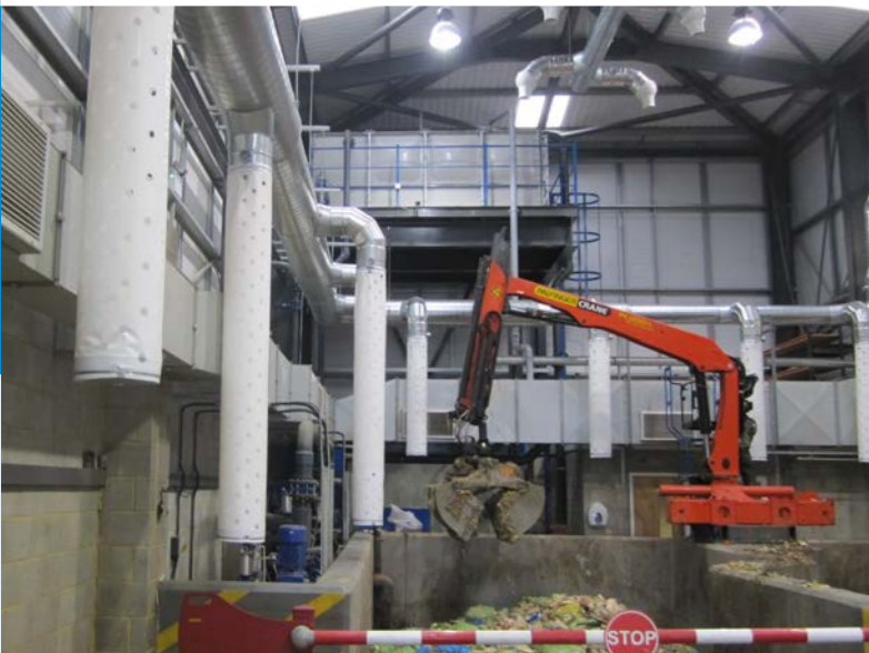
▼ Terminodour™ treatment on a food waste AD plant, England
