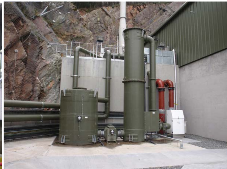
▼ Catalytic iron filter with carbon odour control system at Dunoon WwTW for Scottish Water
