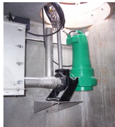
▲ Pump mounted on a guide rail for Easy above chamber maintenance
