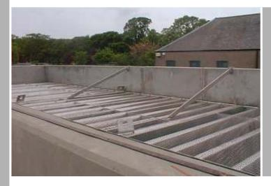
The channel shown above was lifted into the storm storage chamber after the screens had been attached to the concrete overflow.
