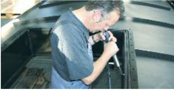
Draw welding on a PE-container with the DIODE PID.
