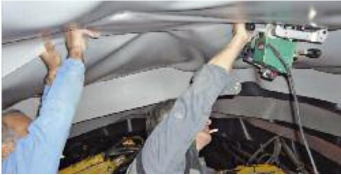
Comet operating in the tunnel ...
