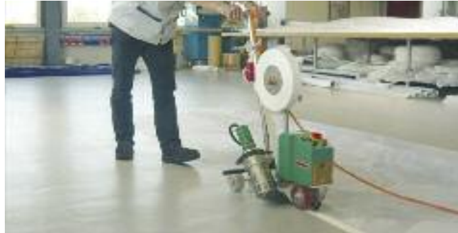
Welding tape at maximum speed.
