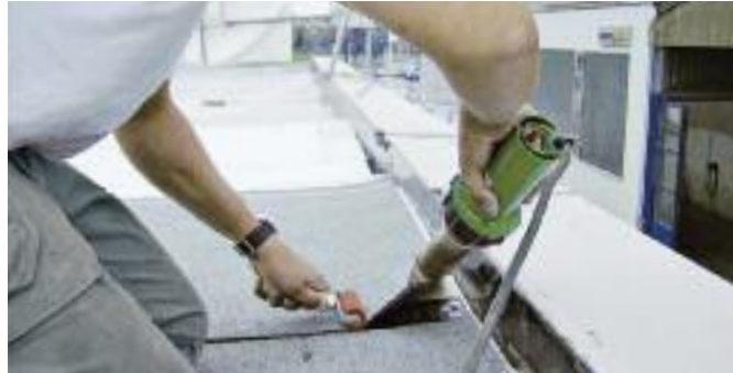
Welding of bitumen sheeting using the powerful ELECTRON with a wide slot nozzle.
