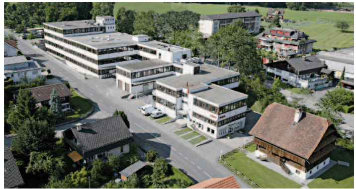
Leister Technologies AG, production building, Kaegiswil, Switzerland
