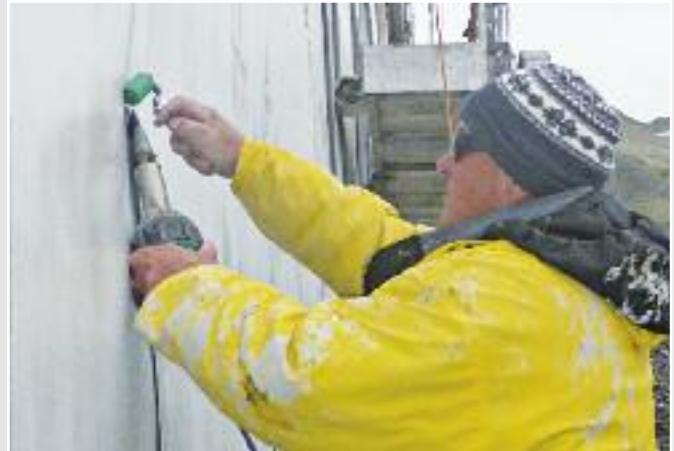
A specialist produces perfect welding seams using a reliable TRIAC S.
