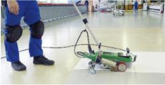
Constant, wrinkle-free overlap welds.
