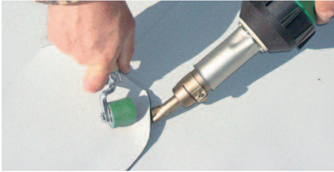
TRIAC S while overlap welding on the roof..
