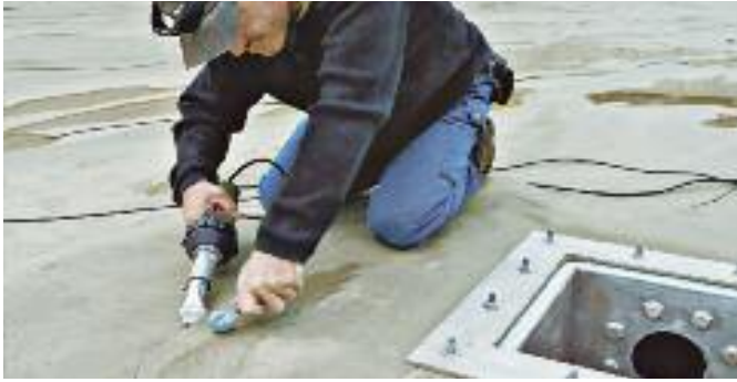
TRIAN S in use welding a future a storage reservoir.
