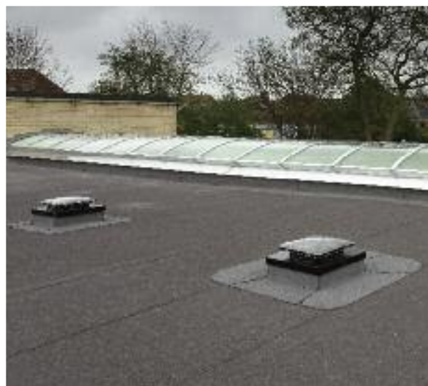
Em-Tube with PVC 150mm upstand on flat roof
