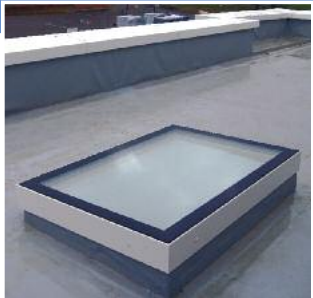
Em-Glaze Modular to builder's upstand
