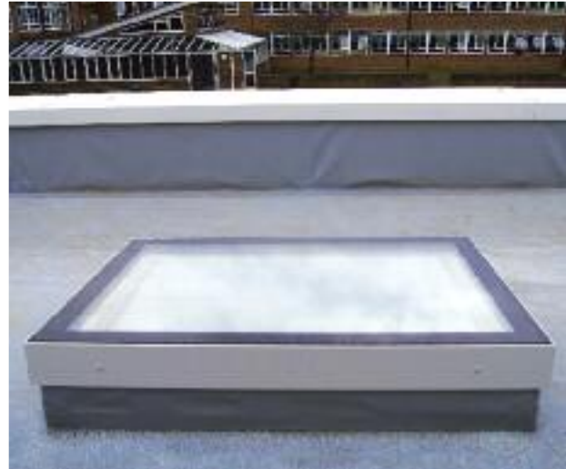
Em-Glaze Modular to builder's upstand
