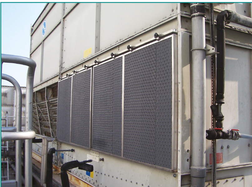
Following completion of removable Crossflow fill pack kit
