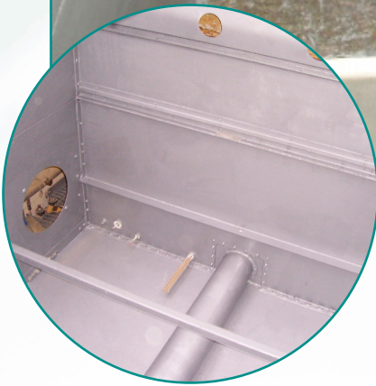
Surface preparation for high performance paint system
