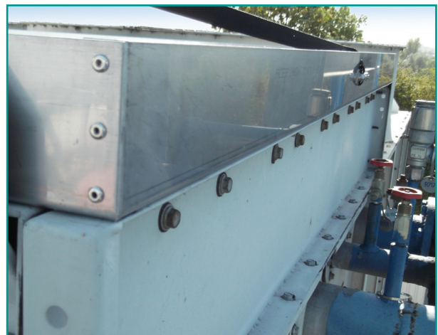
AFTER: Tower Systems installation with stainless steel support frames and retention strapping.
