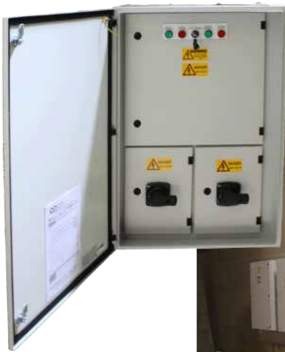
Combination ATS with external door open
