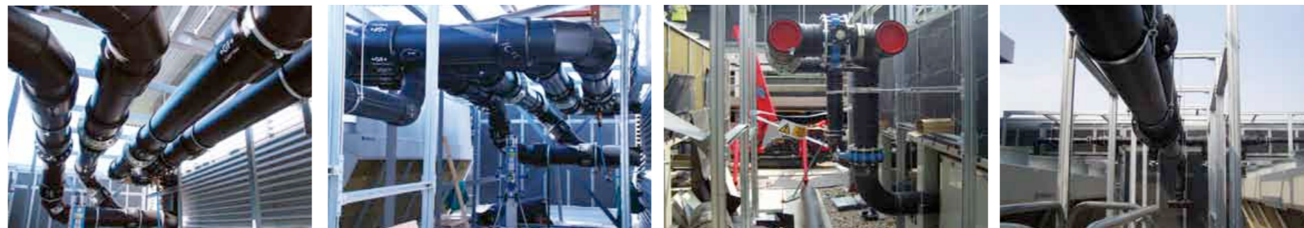
Fabricated assemblies delivered directly to site
