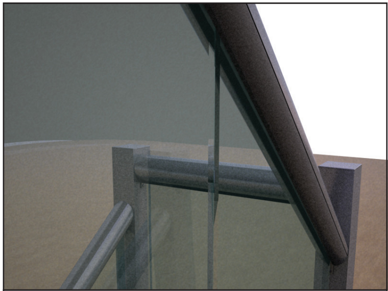
42 Hand rail full length glazing bead into position
