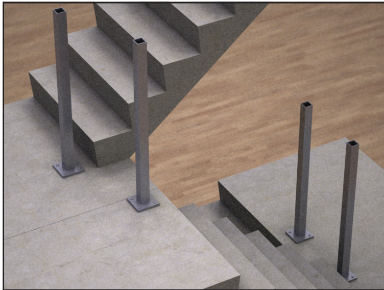
7 Fix the post firmly to the structure making sure they are perfectly vertical
