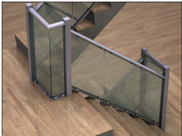
36 Make sure that all the glass panels are properly aligned
