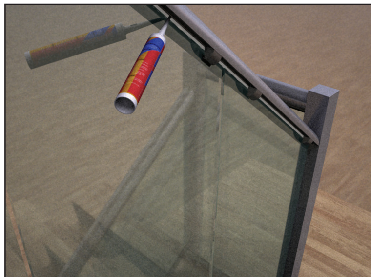
38 Apply a thick bead of high quality silicone sealant to continuously fill the gap between bottom of glass and bottom rail
