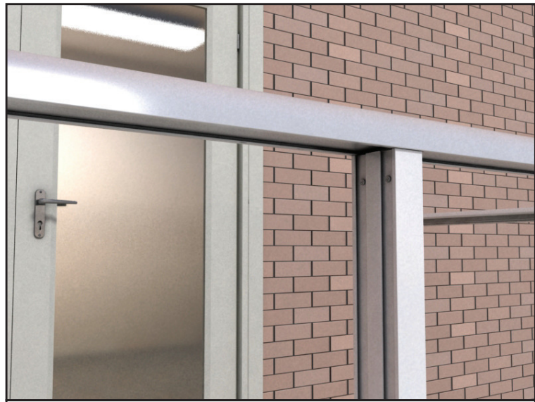
30 Fix the post into the post connector the No. 8 x1/2" S/tapping screws provided
