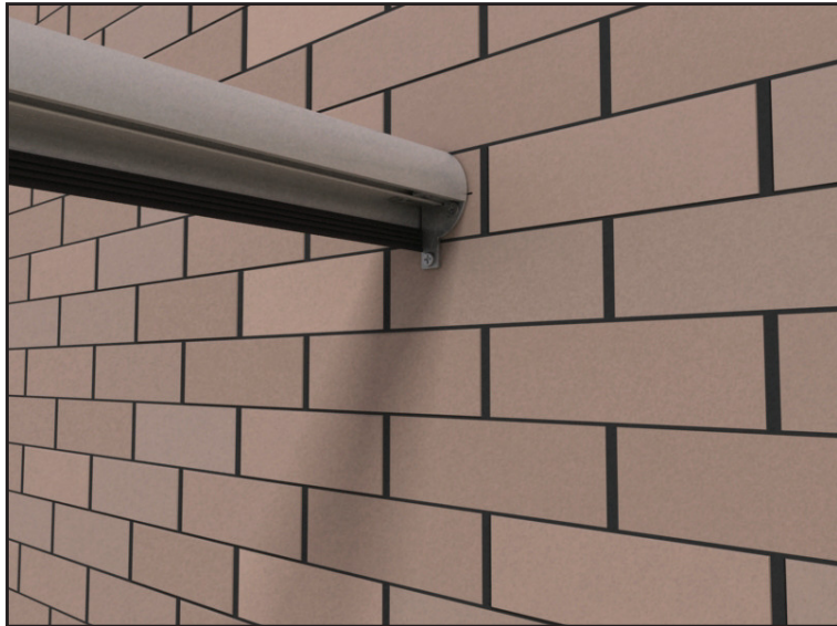
26 Drop the handrail onto the angle bracket
