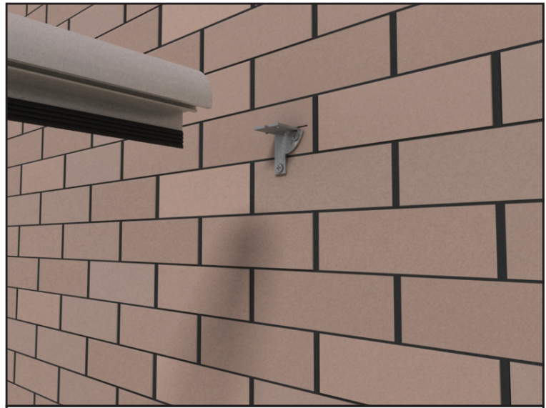
25 Bring the handrail into position
