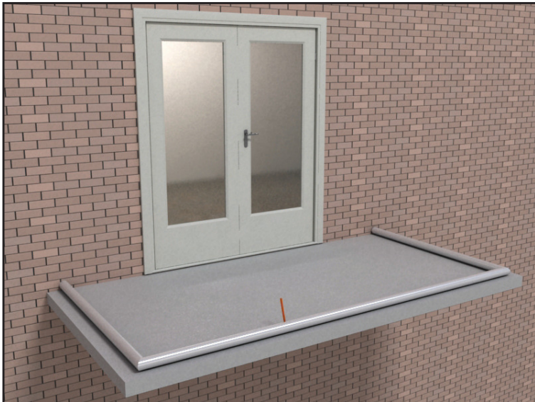
13 Place handrail on the floor in position to make sure the dimension and shape fit
