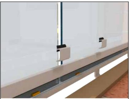
14. When the silicone is dry, replace the small glazing beads with the full length glazing beads top and bottom.
