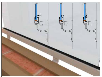
15. When the full length beads are in place push in the 3mm rubber gasket between the glazing bead and glass, soap and water can help.
