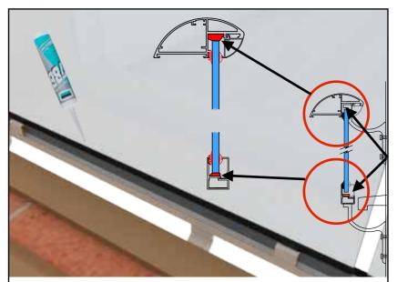
13. Using silicone, fill the space between the bottom of the glass and track and between the top of the glass to the underside of the handrail. Do this along the entire length, top and bottom.
