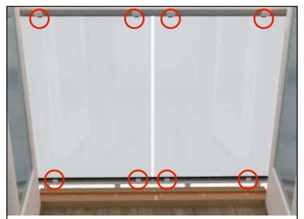
11. Place the glass panels in their positions. To hold them temporarily in position use the small glazing bead pieces provided and 3mm rubber in the handrail and the bottom track.
