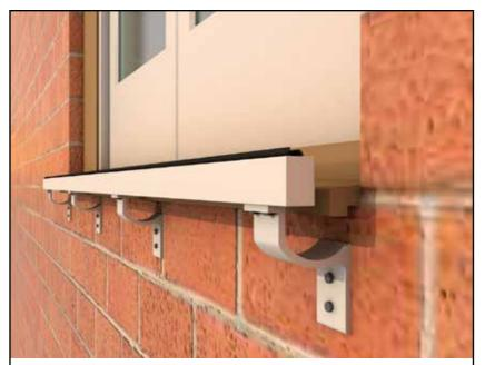
3. When properly lined up, fix the bottom track brackets firmly to the wall. (Use a level to make sure it is horizontally level.)
