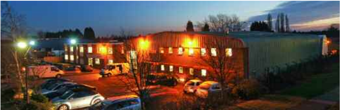
TOP-TEC design and manufacturing headquarters Birmingham, England
