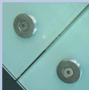
Special order - vandal proof panel fixings in stainless steel, holding glass panels to wall.
