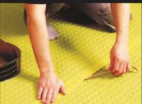
DELTA<sup>®</sup>-FM specifically is designed for floor applications, to combat dampness, and contamination. The special low
