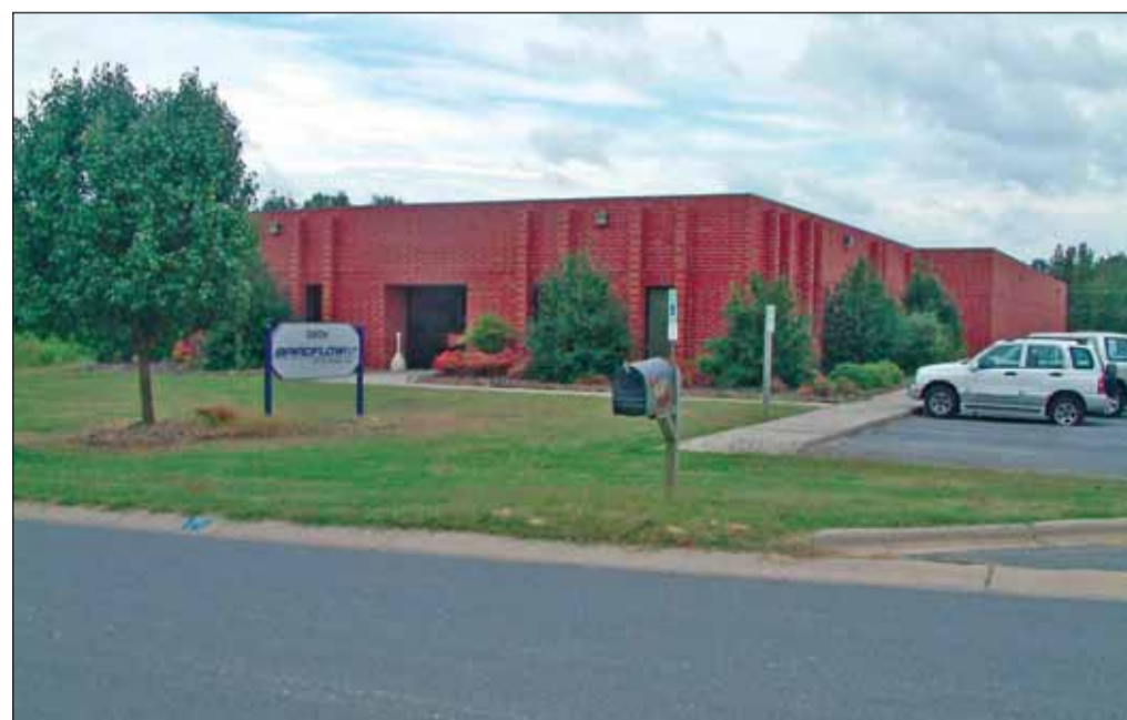
The Charlotte, North Carolina, factory and administrative offices of Spiroflow Systems, Inc.
