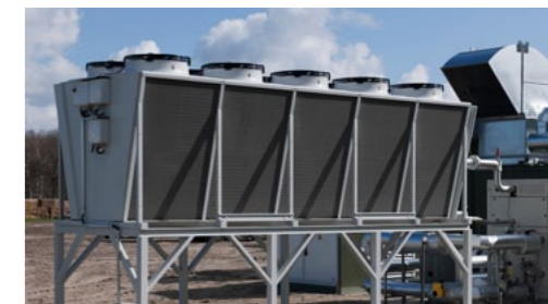
The Güntner condenser GVD, specifically developed for the energy industry, cools the working fluid used in the ORC process.
