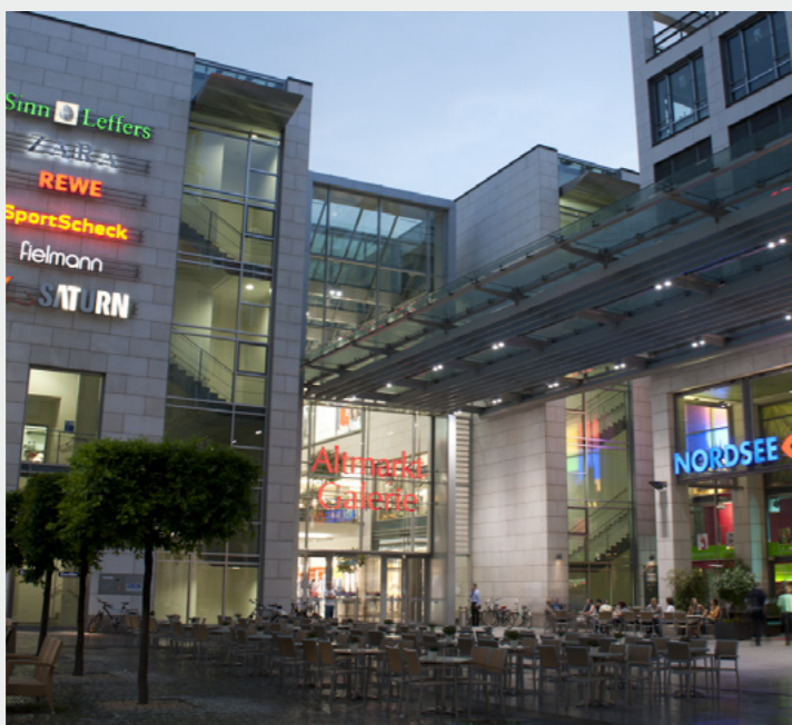
5 Efficient air-conditioning: drycoolers equipped with EC fans save 92,800 kWh per annum.
