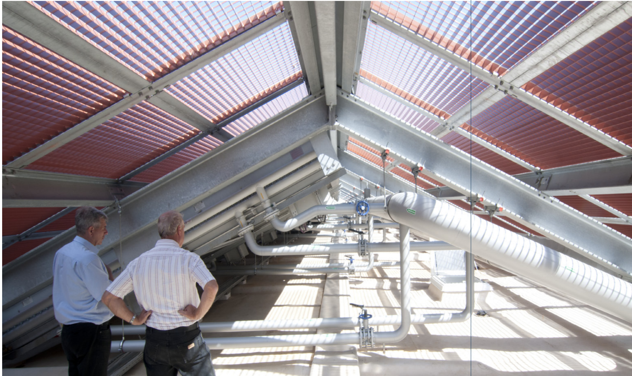
View of the drycoolers after installation of the sight screen
