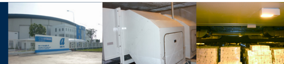
The evaporators are provided with service hatches for easy access to the fans
