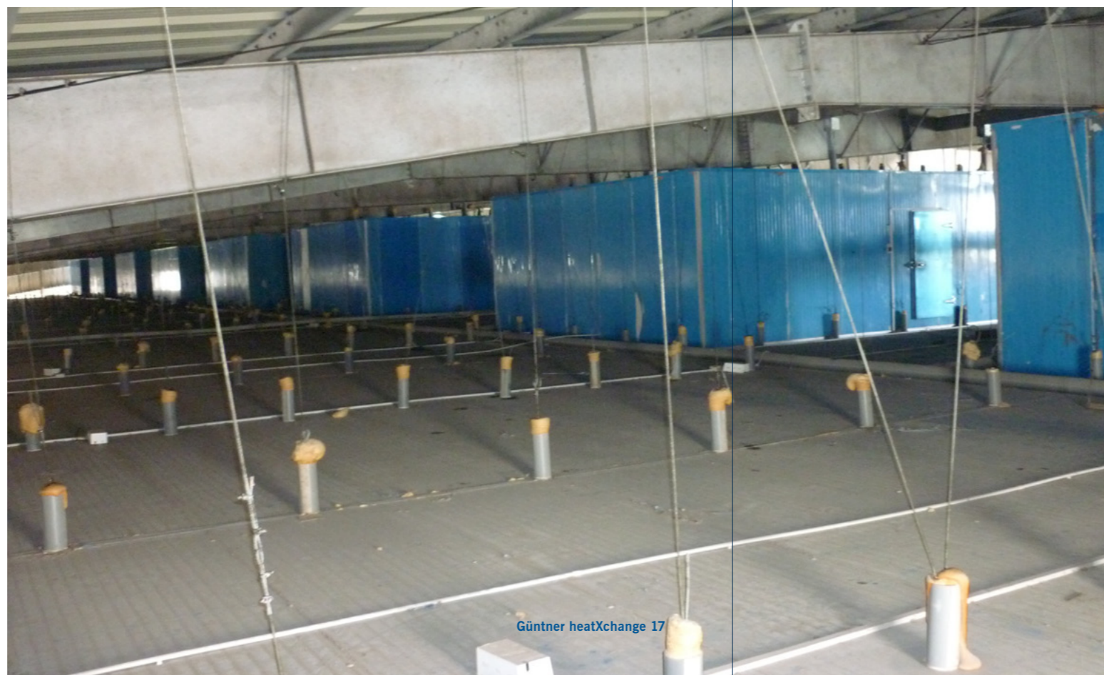
The penthouses are located on the roof of the insulated cold storage facility, underneath the protective pitched roof.
