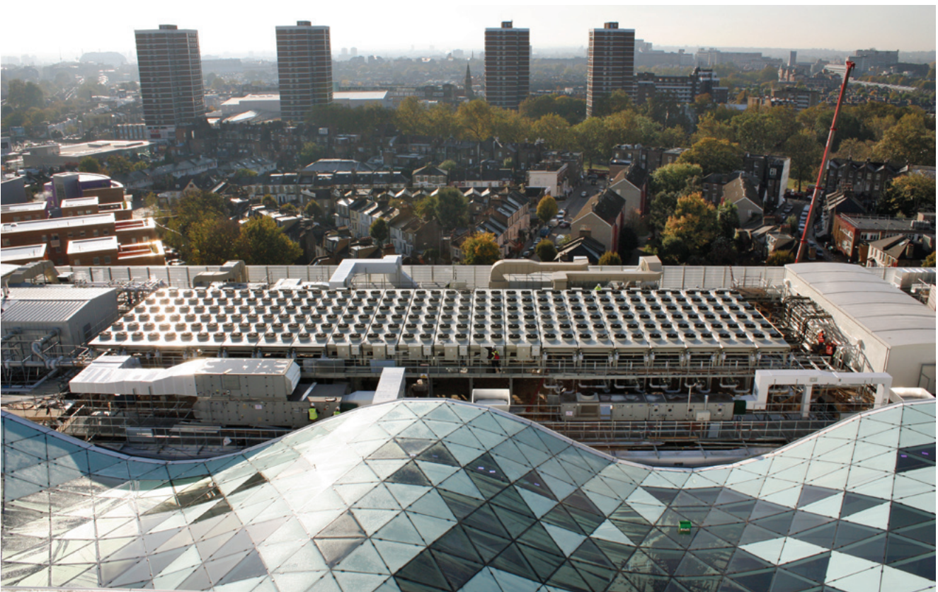
The drycoolers operate in a low-noise mode.
