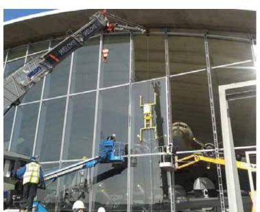
Duxford Imperial War Museum required a specialist contractor to undertake works on the Sir Norman Foster designed American Air Museum Hangar. Working alongside a Principle Contractor, Glazing Refurbishment were instructed to conduct the removal, repair and reinstatement of the existing curtain wall system.
