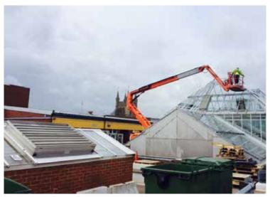
Working for Savills UK, Glazing Refurbishment submitted a phased refurbishment program for Kennett Shopping Centre to refresh the existing glazing systems and return them to a serviceable standard. The Centre has suffered from a lack of maintenance which had resulted in a number of defective panels and numerous leaks throughout.
