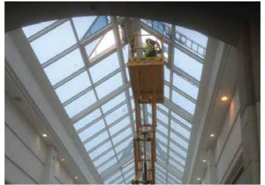
The new owners of the St Elli Shopping Centre inherited an overhead system with multiple water ingress issues due to the seaside location and a lack of maintenance.
