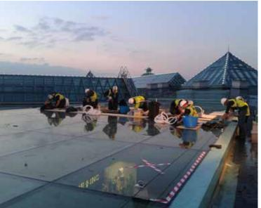
Having experienced water ingress issues with a recently installed overhead rooflight measuring over 100m in length, we were tasked with inspecting the system and providing a long term solution.
