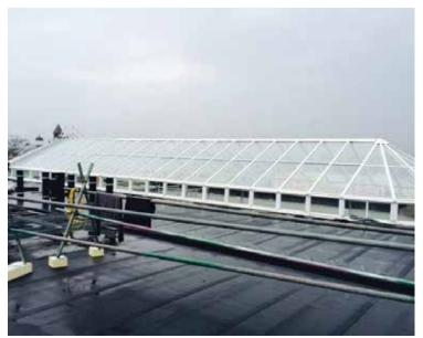
Spires Shopping Centre required a full refurbishment of the existing glazed mall/atrium. This large scale operation involved the complete removal and disposal of the existing glass units and system components.
