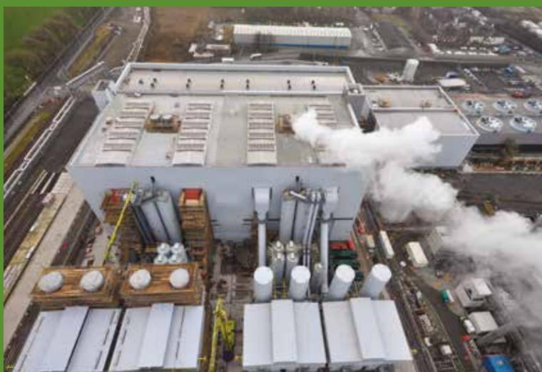
▲ The EfW at Runcorn in February of this year. The site has been undergoing a commissioning process, including a steam-blowing procedure
