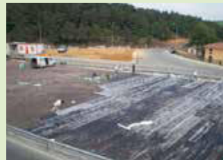
Floor slab waterproofing
