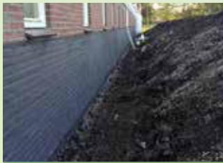
External basement waterproofing
