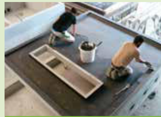
Precast concrete production
