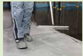
Coating after 24 hrs
