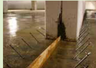
Water-bearing joints
