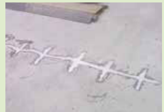
Crack stitching
