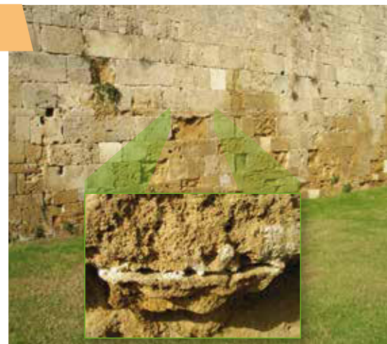
Salt crystals on the surface
