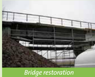
Restoration of support beams
