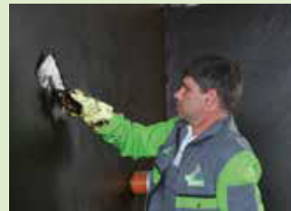
Waterproofing against Radon
