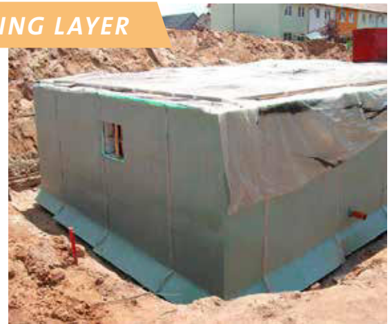
KÖSTER SD Protection and Drainage Sheet 3 - 400
