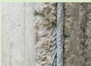
Corrosion protection (coating)
