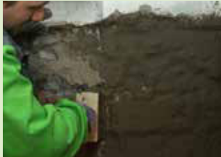
Internal basement waterproofing
