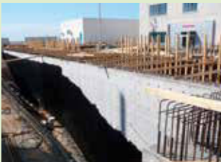
External basement waterproofing
