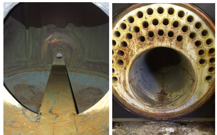
Internal images of the calorifiers prior to removal
