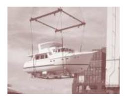
A spreader might be designed to lift a load such as a vehicle or boat, lifting it from the base but keeping the slings clear of easily damaged areas.
