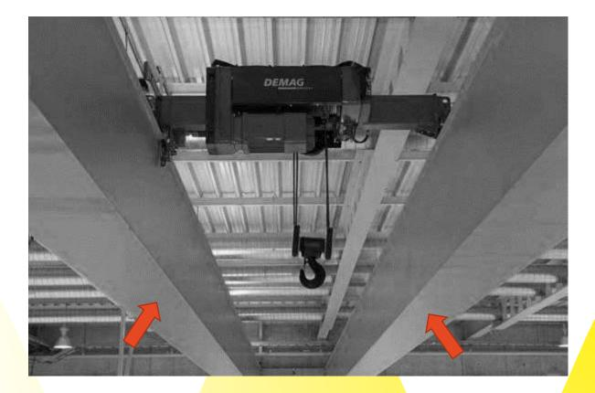
This will allow the lifting beam to foul the girders before the limit switch operates. Adjustment of the limit switch or a secondary operational limit is necessary. Relying on the operator is not good practice.
