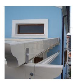
Front profile bracket Joins the arms securely to the front profile and permits adjustment of the angle.
