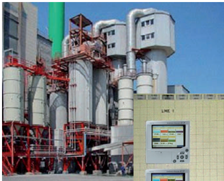
Monitoring and recording system Process control in recycling reactors.
