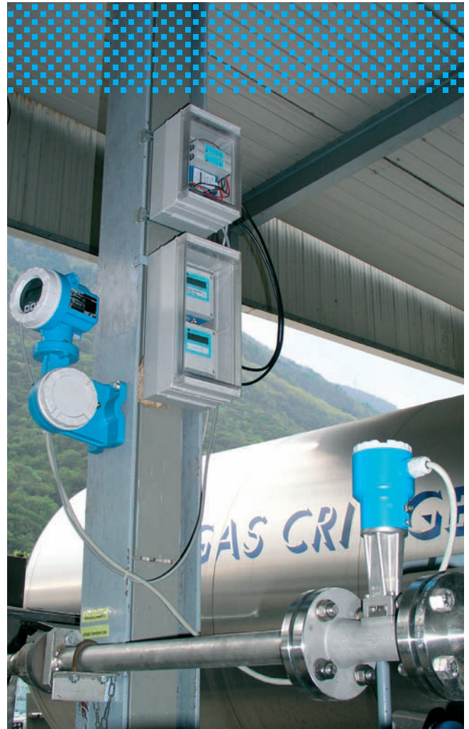
2 Minilog B devices for level measurement and dosing.
