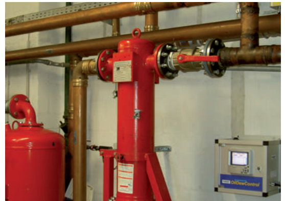
Oil content and pressure condensation monitoring with Ecograph T (OilDewControl). The data is recorded, are traceable and free from manipulation. The user can follow the plot on line from his desk. The installation was done at a food manufacturer in accordance with the new hygiene laws.
