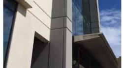
Sandwich panels combine an internal structural leaf with a layer of insulation complemented by the Thermomass system and an external leaf thus replacing the traditional cavity wall system.
