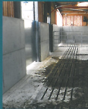
Slatted channels in cubicle house.
