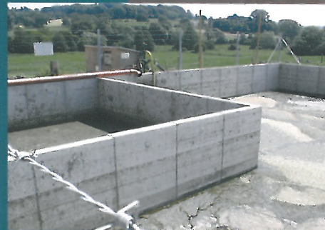
Vertical cantilever panels are the solution for liquid slurry storage.
