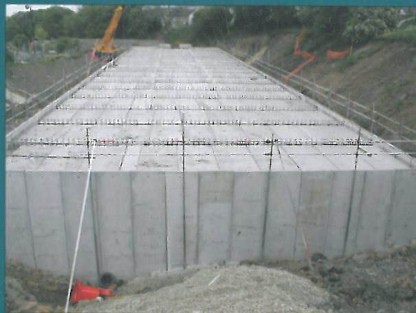
Precast column and beam roof supports with R35 wall panels
