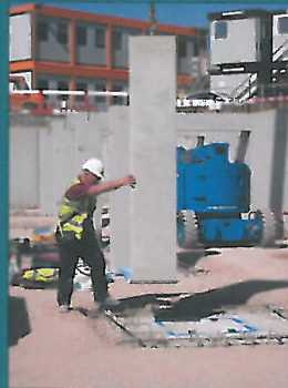
Below ground liquid storage tank constructed with R35 wall panels and precast roof.
