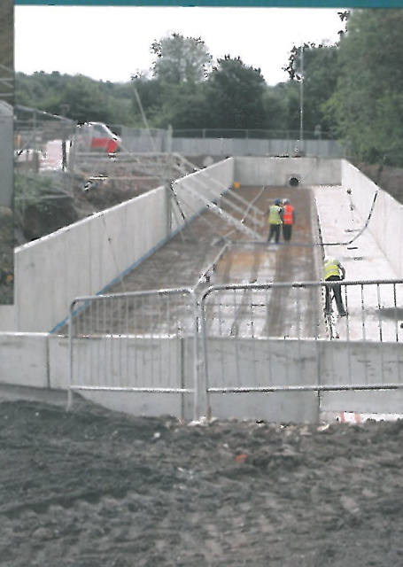
Installation of prestressed vertical cantilever panels
