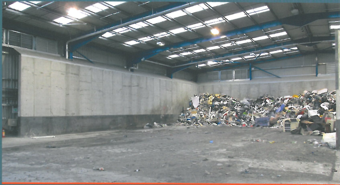
Push Walls 5m high - 280mm thick vertical cantilever prestressed concrete panels.
