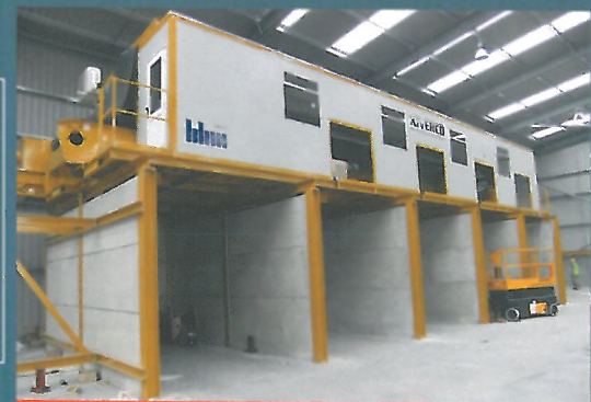
Concrete panels are ideal for recycling bays and picking stations being low maintenance and robust.
