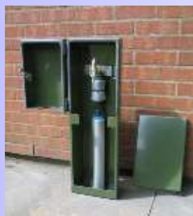
Lower Access Panel Can be removed for installation & service access
