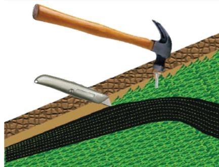
Trim the edges to shape using a sharp Stanley knife, remember to cut through the backing of the grass first. Secure the grass to the timber batten using galvanised ring shank nails every 15-25cm.
