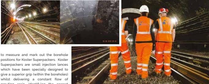
grouting resin. Identifying the correct injection packer placement is an important process. Koster specified the Injection ports to be placed at 400mm centres in a grid pattern, with a single packer positioned in the centre.
